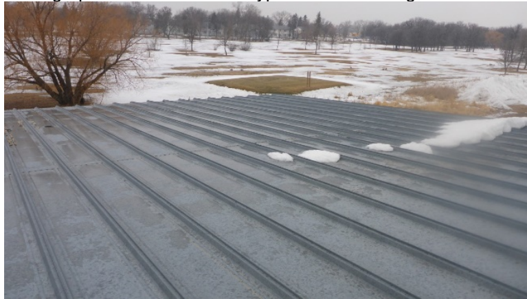
Photograph 5.3.2.3-1: R3 roof type. Metal standing seam roof.
