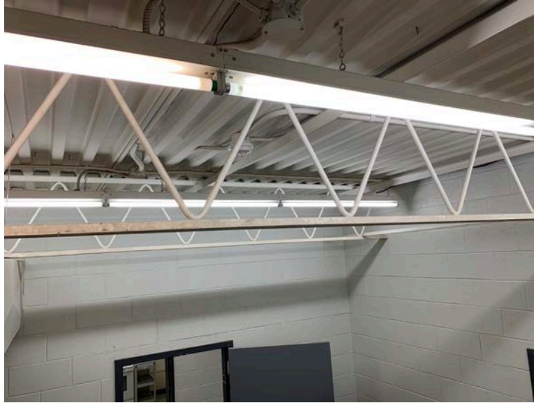
Photograph 3.2.2.4-1: Steel joists at low roof.
