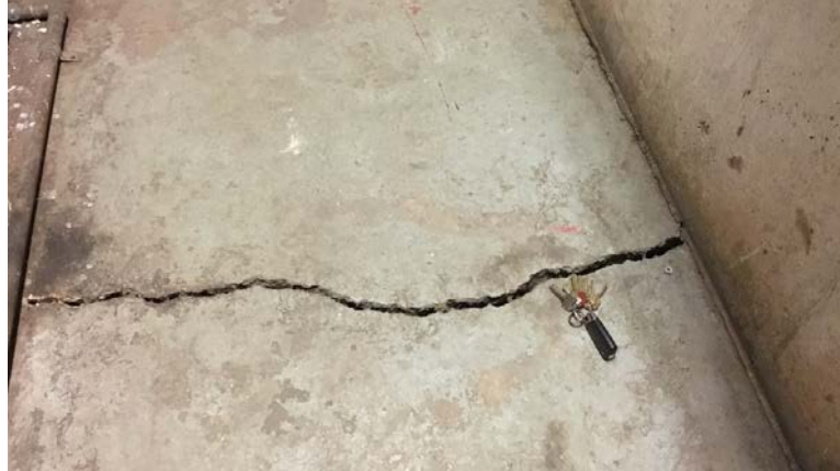
Photograph 4.2.1.3-1: Partial view of basement slab scaling.
