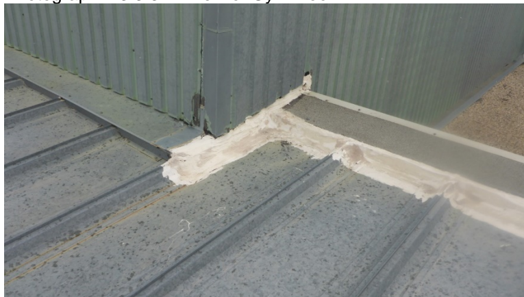
Photograph 4.3.3.3-1: View of Gym Roof R4.
