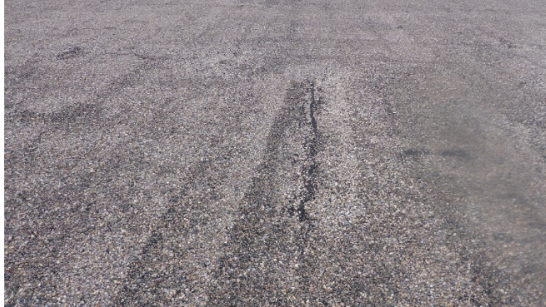
Photograph 5.3.2.1-3: Typical exposed asphaltic membrane.
