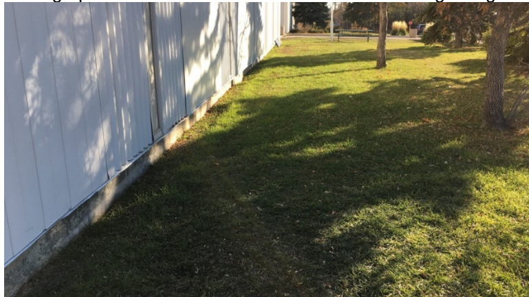
Photograph 4.1.2.2-1: Partial view of south elevation grading.
