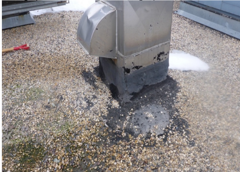
Photograph 4.3.3.2-3: View of existing repairs.
