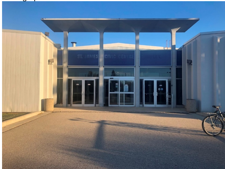
Photograph 4.3.1.3-1: Over-all view of the main entrance at the St. James Civic Centre.
