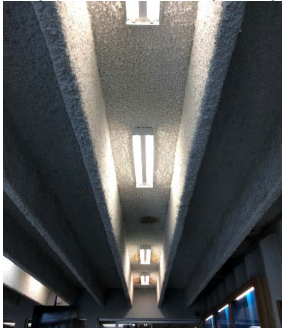
Photograph 3.3.1.6-1: Water staining on ceiling at light fixture locations.
