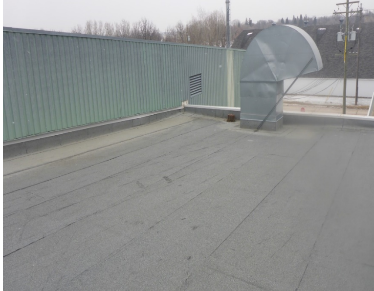
Photograph 4.3.3.1-2: View of upper roof facet R6.
