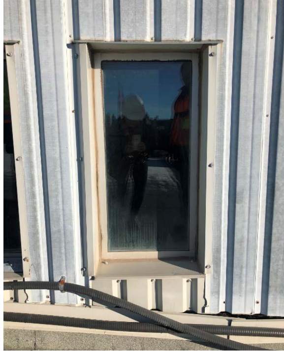
Photograph 4.3.2.3-1: Typical second story aluminum framed window.
