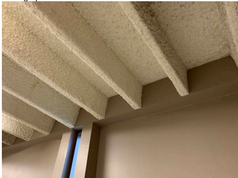
Photograph 3.2.2.3-1: Precast concrete roof tees.
