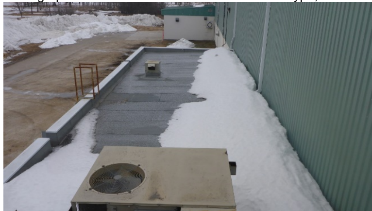
Photograph 5.3.2.2-1: SBS modified bitumen roof type, R2.
