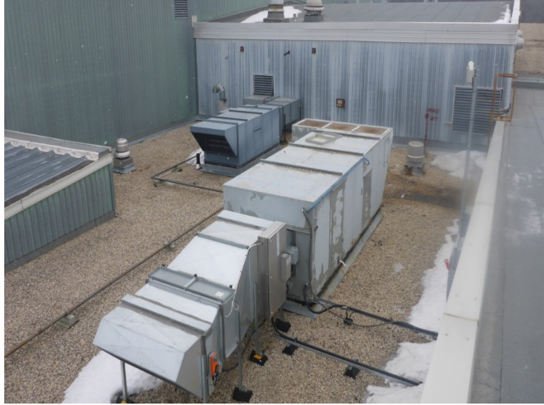
Photograph 4.3.3.2-1: Showing lower roof R5.
