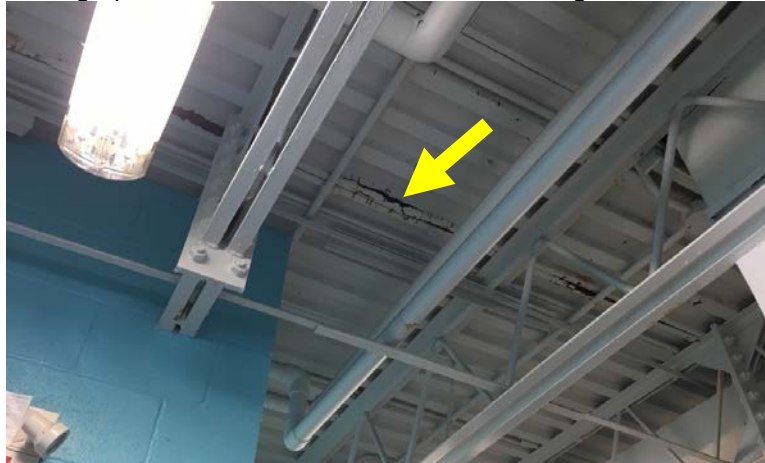
Photograph 4.2.4.1-3: Partial view of roof framing.
