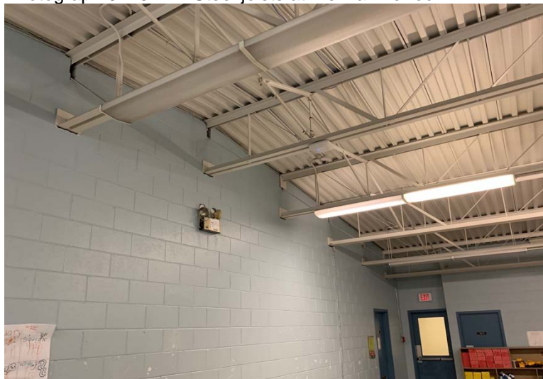
Photograph 3.2.3.1-1: Steel joists at mezzanine roof.
