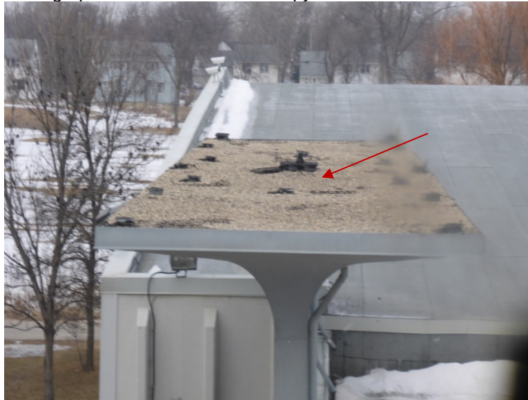
Photograph 4.3.3.2-2: View of canopy roof R12.
